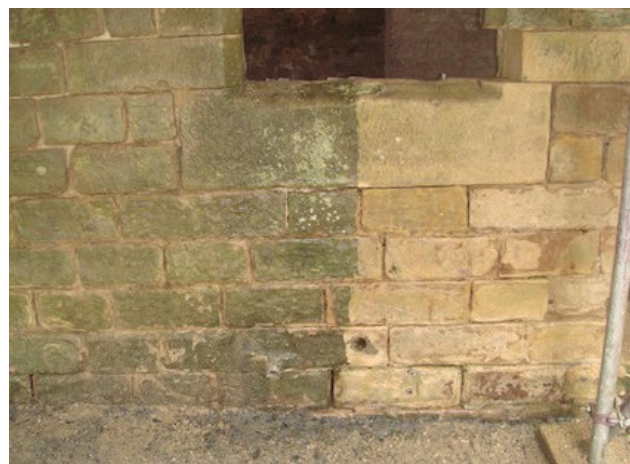
Algae and lichen being removed from a stone building using a low-pressure steam based system.
