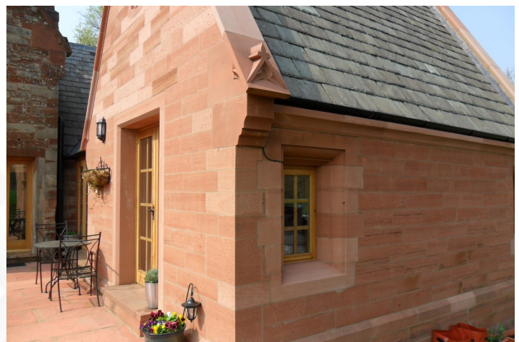
An Ashlar Extension with Profiled Window Surround Stones and a Profiled Kneeler Stone below the Gable Copings
