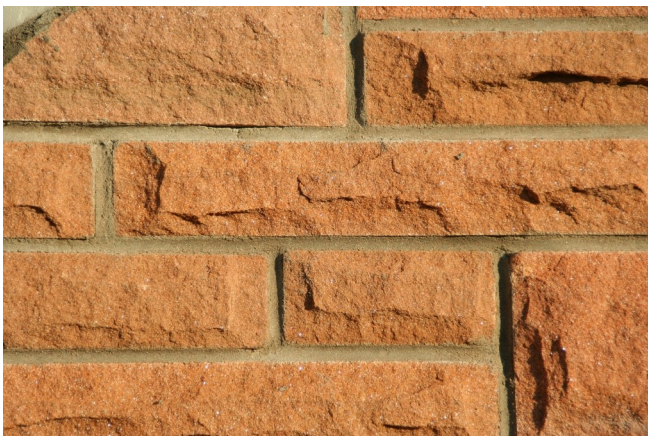
Red Sandstone with a Cement Mortar Construction
