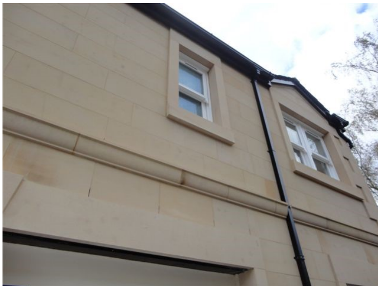
An Ashlar Façade with a Feature Profiled String Course
