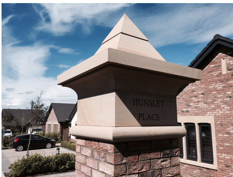
A Splayed and Profiled Pillar Cap With a Bullnosed Collar Detail and V-Cut Lettering
