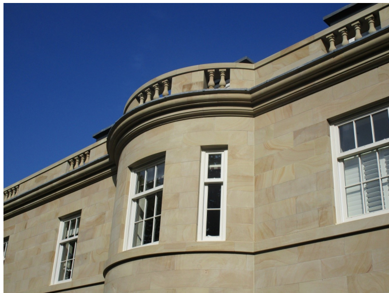
An Ashlar Façade with a Feature Cornice and Band Course
