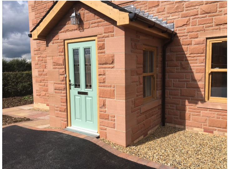
A Pitched Walling Porch with Smooth Quoin Stones
