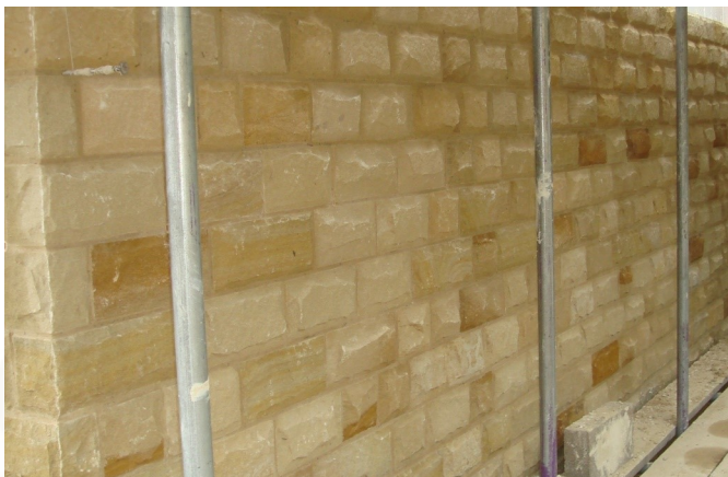
Buff Sandstone With a Lime Mortar Construction
