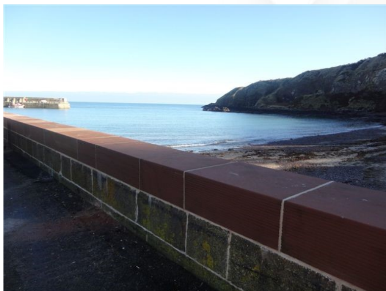
Large Sandstone Copings to a Harbour Wall
