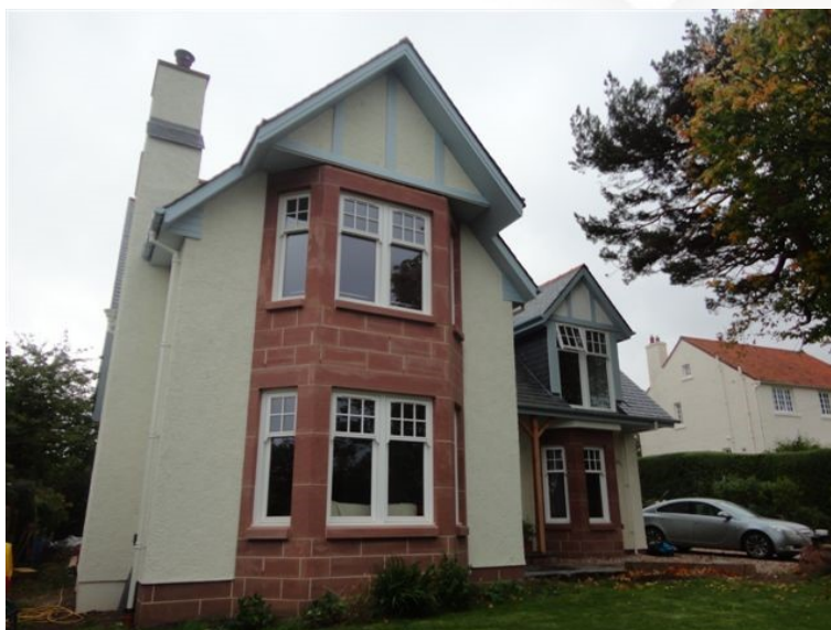
A Red Sandstone Bay Window with Angled Mullions
