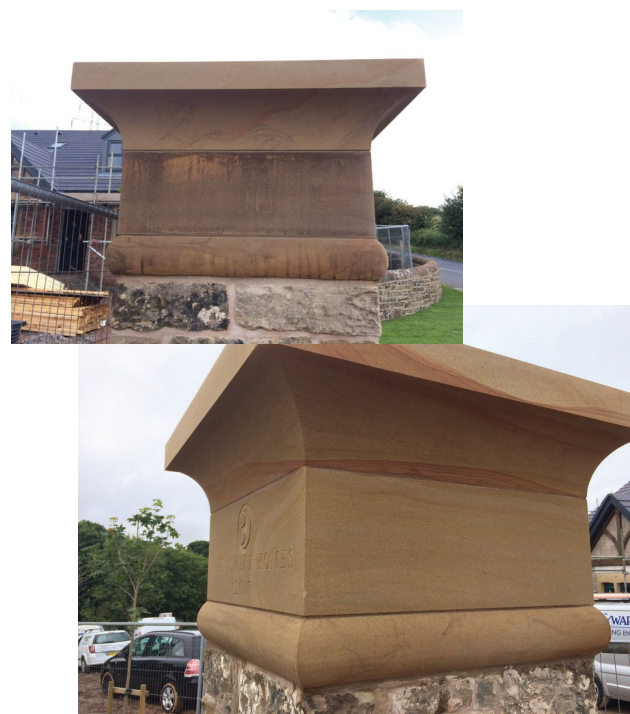
A sandstone pillar cap before and after cleaning. A chemical was applied to the stone to remove the black discolouration that had started to appear.
