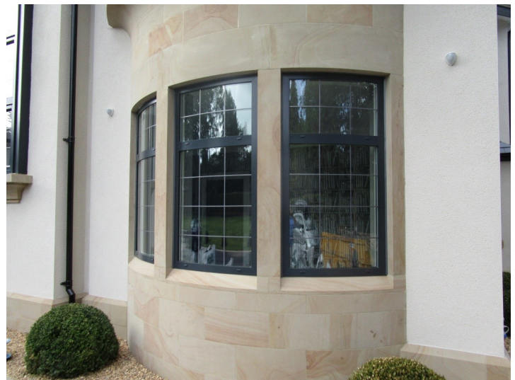
A Radiused Bay Window with Central Mullions
